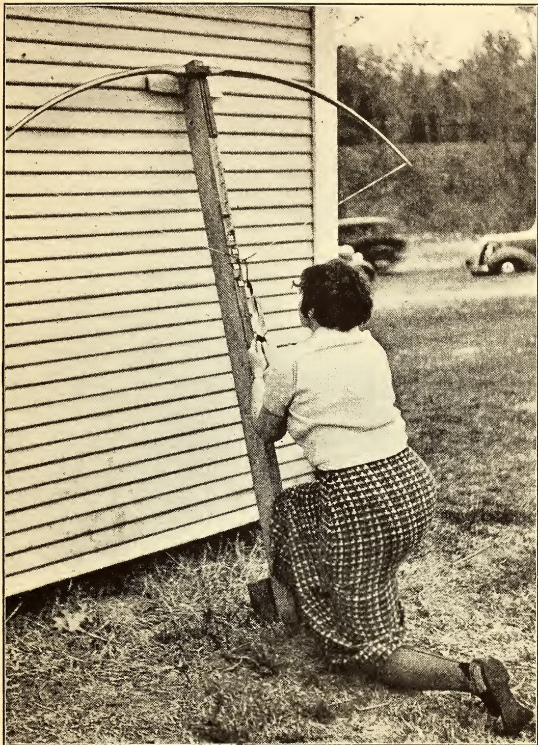
(2) A DEVICE FOR TESTING BOW WEIGHTS
